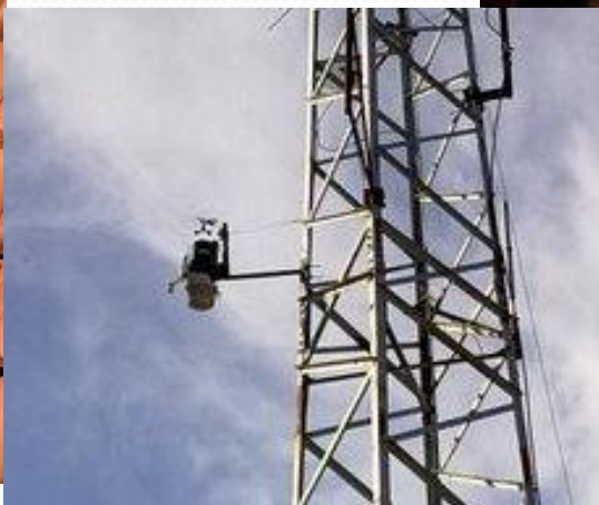
Meteo station and internet
